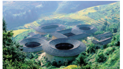
Hakka-Lehmhäuser in Yongding
